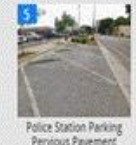
Police Station Parking Pervious Pavement
