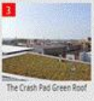
The Crash Pad Green Roof
